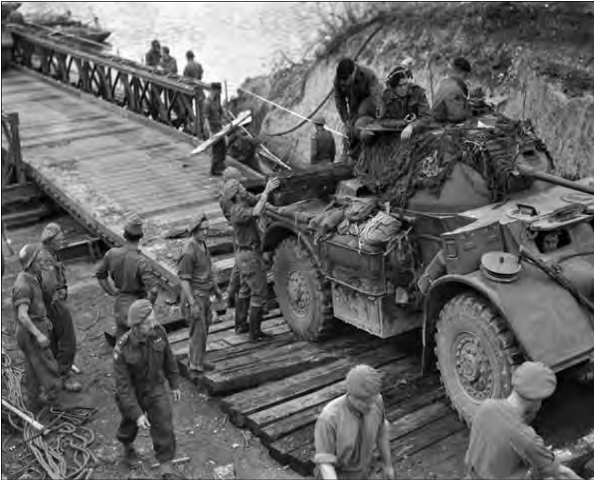
British Engineers setup a Bailey Bridge – Gothic line Eastern Sector
