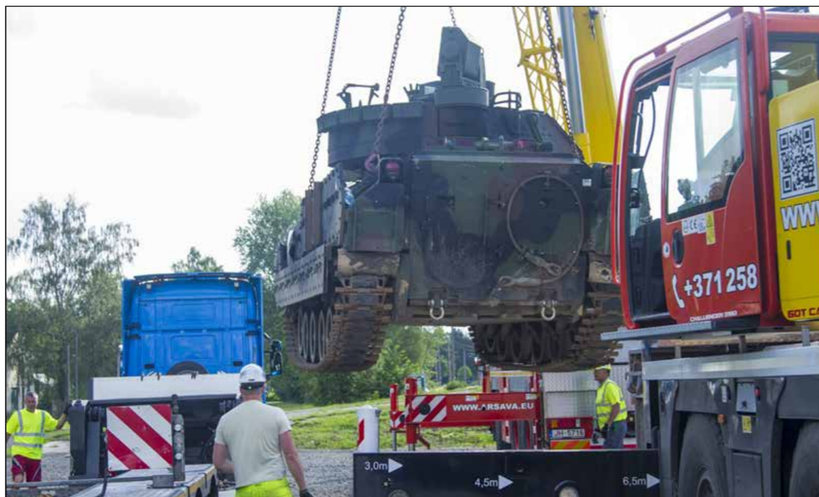
Fig. 3: Contractors move a Bradley M2A2 off a rail flat.
